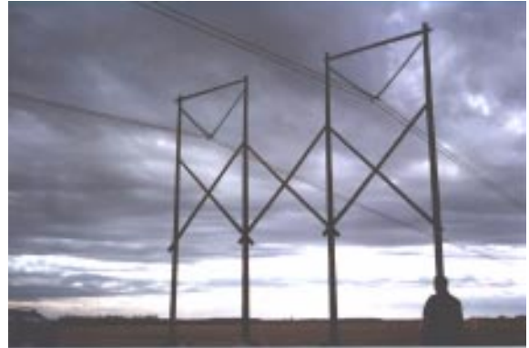
Fig. 2 Temporary Wood Pole +/- 500kV DC
